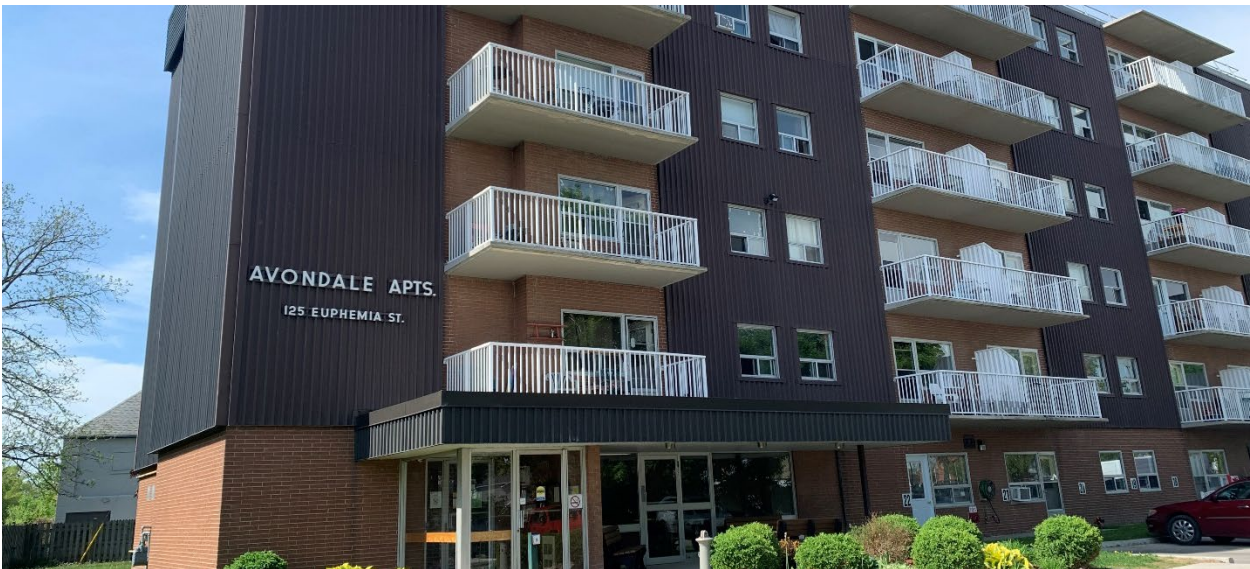
IMAGE: The Avondale Apartment Building in Sarnia
